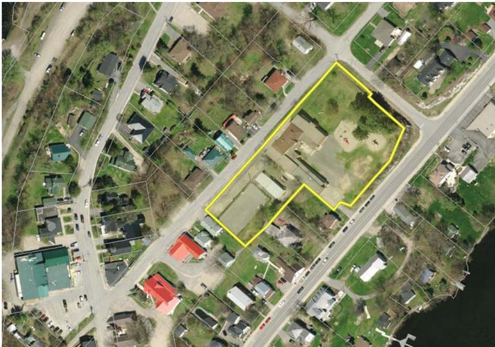
Figure 4 – Garrett Street site (Sharbot Lake P.S. property)
